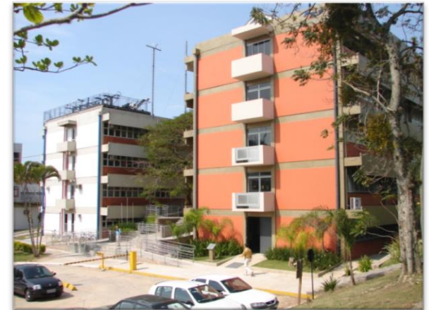
Buildings A1 and A2
